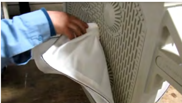
Click to Watch Video: "How to Install a CGR Filter Cloth"
